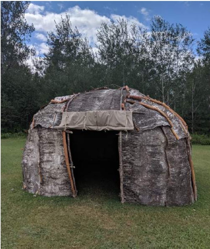
Waaminogaan built from iron wood and birchbark by Russel Northrup and Family in August 2019
