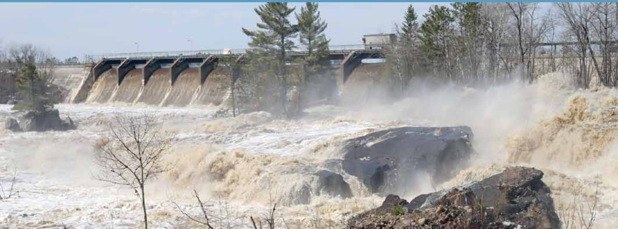
The Thompson Hydro Station on the St. Louis River as rapidly melting snow brings water surging from the dam and over the rocks.
